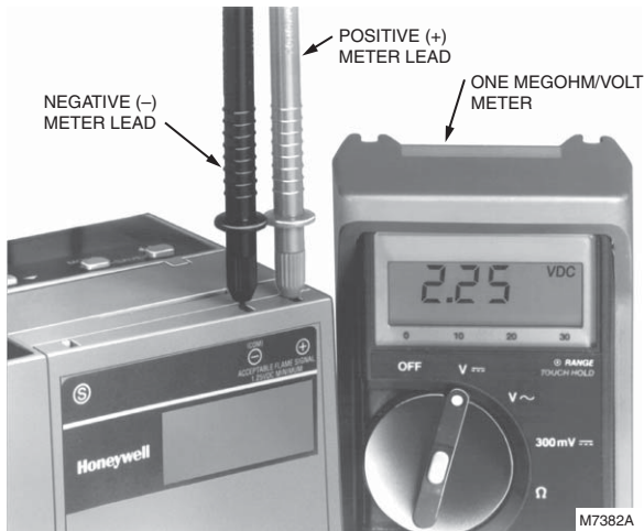
Fig. 11. Measuring flame signal voltage of 7800 SERIES controls.
