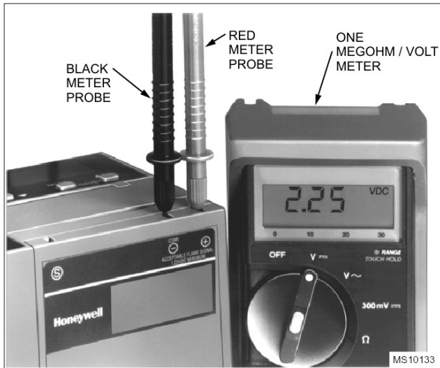
Fig. 11. Measuring voltage flame Signal with 7800 SERIES controls
